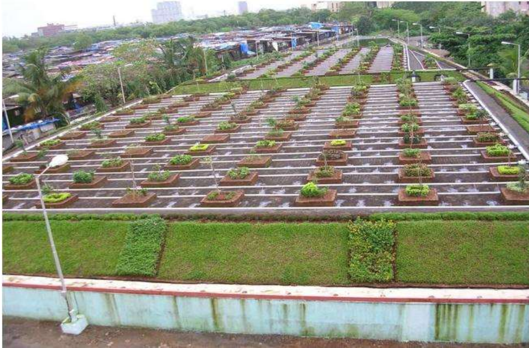
Fig 19.1: 3000 KLD SBT plant in BMC Worli, Mumbai.
